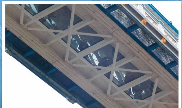
Original steel lattice framework was preserved
