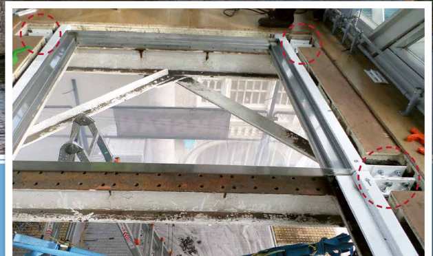
New frame connected by steel fins and support brackets
